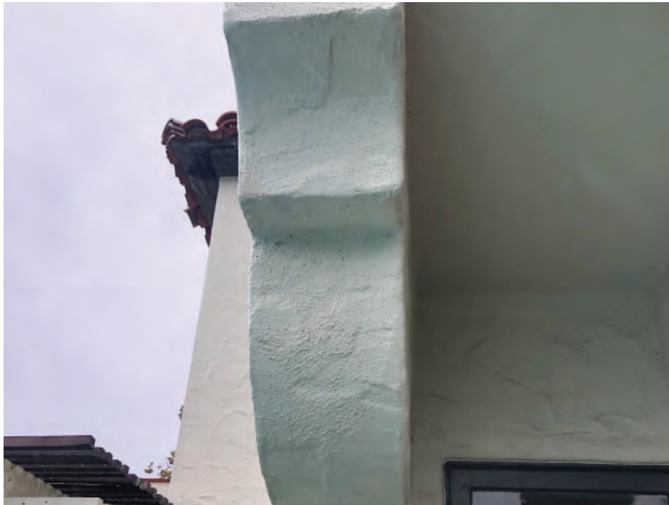
Photo 11: Detail of the curved corner corbels at the northeast facade. Source: John Porter, Home Owner.
