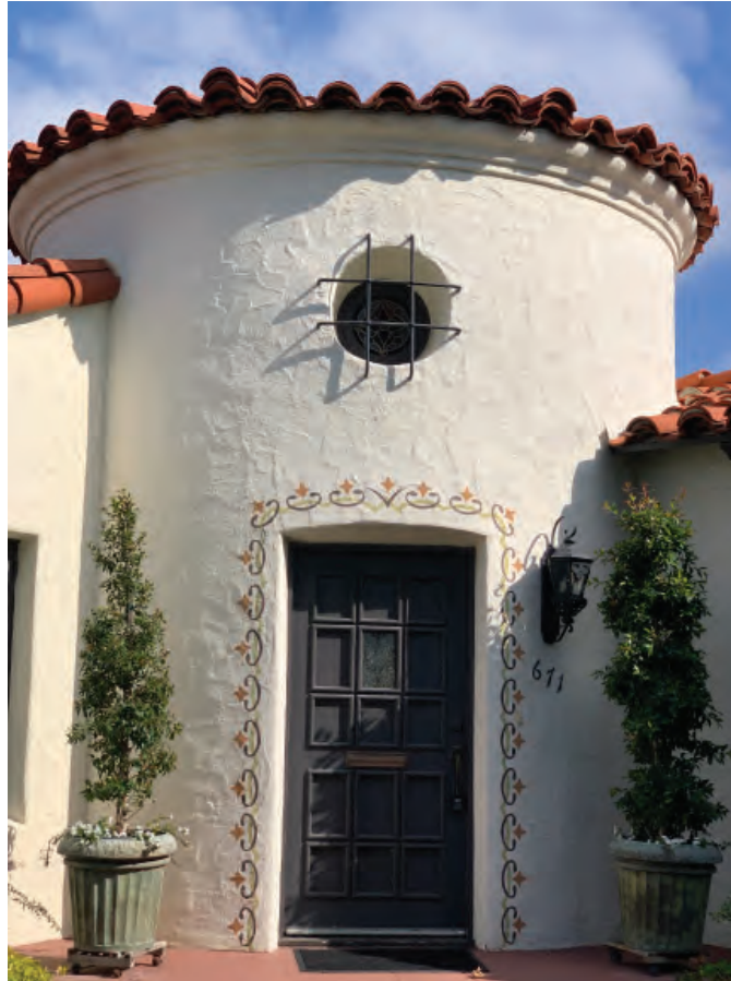
Photo 3: The tiled roof turret corner entry features a recessed entry door with ornamental stencil surround. The entry door is a heavy wood paneled door which replaced the original door in ca. 2000. A recessed porthole stained glass hopper with metal grille is located above.
