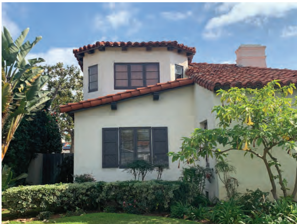
Photo 6: View of the two-story northwest facade. Note the wood, divided lite fixed and casement windows throughout. The tiled roof includes low overhanging eaves and curved rafters.
