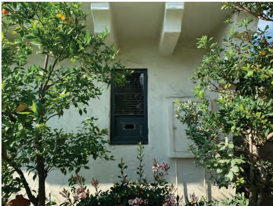
Photo 10: Detail of small casement window at the northeast facade showing through-window air conditioning vent at the lower panel. Note the curved stucco corbels beneath the catelivered second floor.
